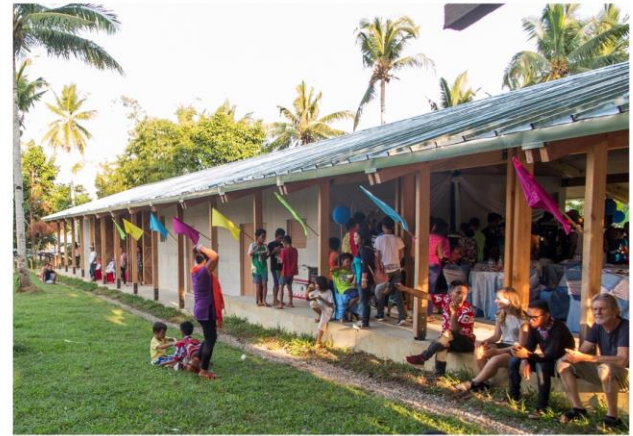
PARK AND PLAY AREA BETWEEN BUILDINGS
